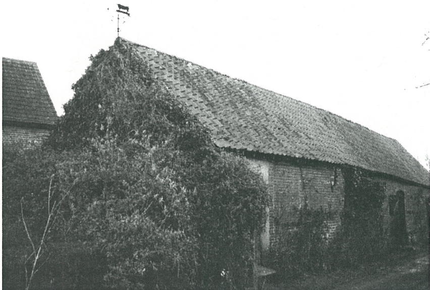
High House Farm (original cottage).
